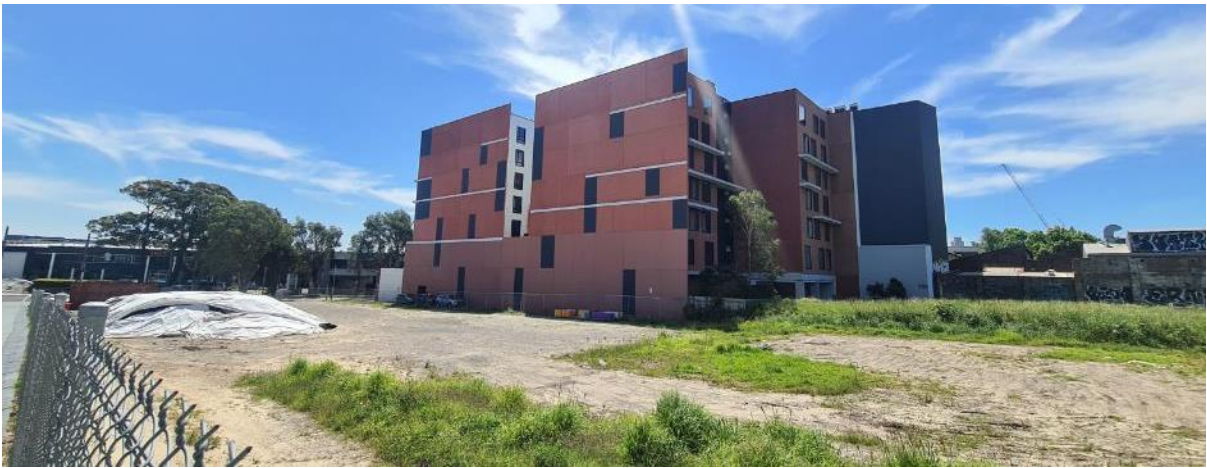
Figure 10: View looking north over the subject site and to the Veriu Hotel at 18 O'Riordan Street
